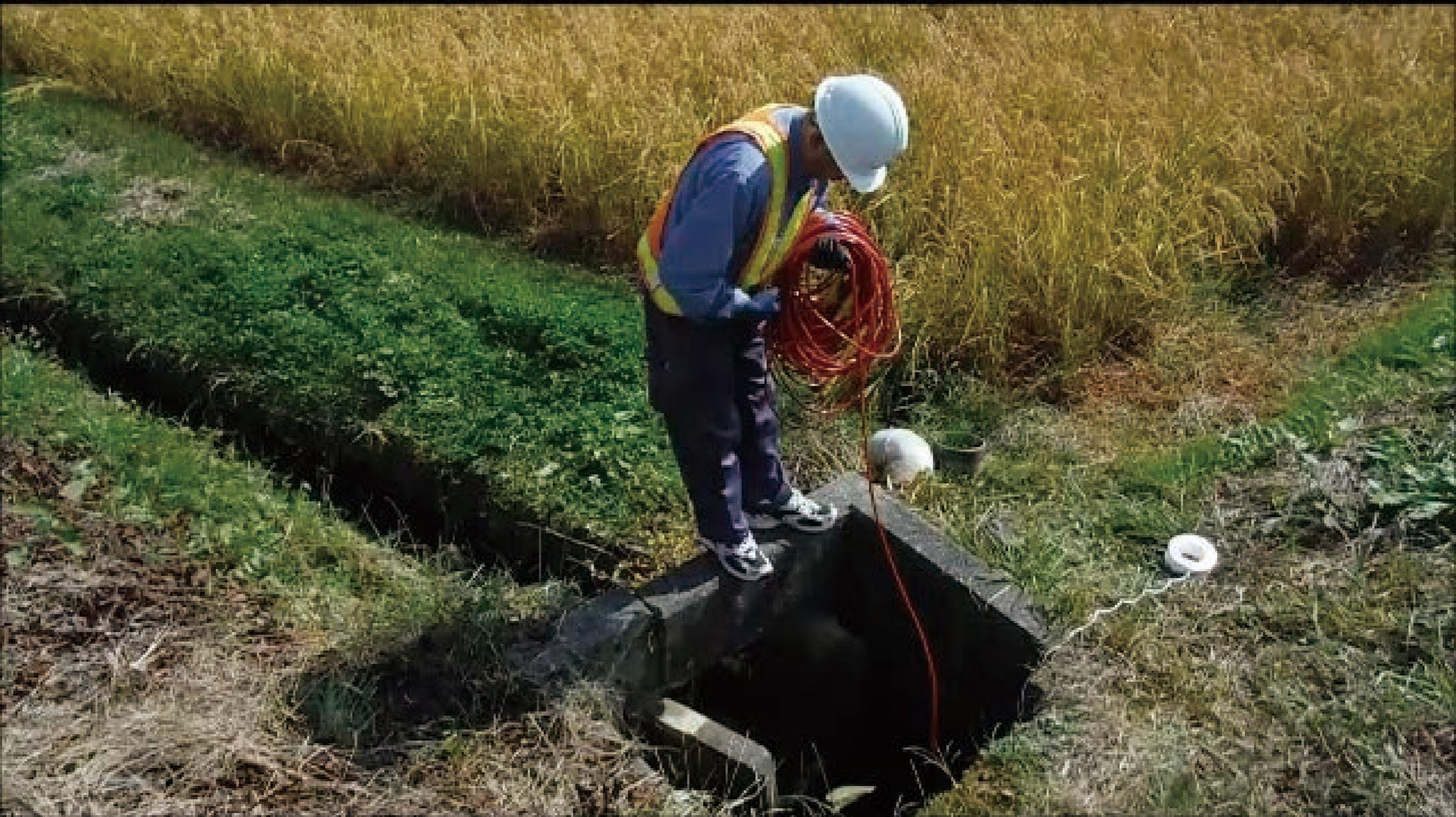
When crossing a road, cable is shown into a drainpipe
